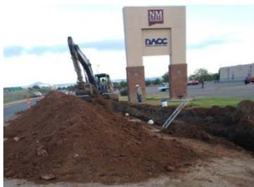
(Left) Also underway is the installation of a 24” diameter domestic water line on the east side of Sam Steele Way from Well 17 to Well 10 is scheduled to be completed in early September.
