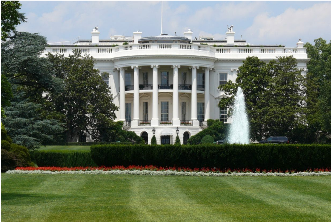
The White House South facade. Wikicommons
